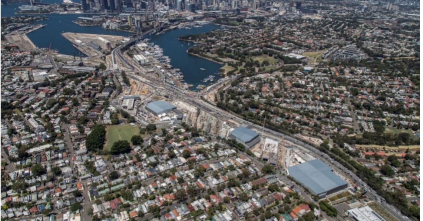
Source: case study and imagery provided by John Holland and CPB Contractors Joint Venture (JHCPB)
